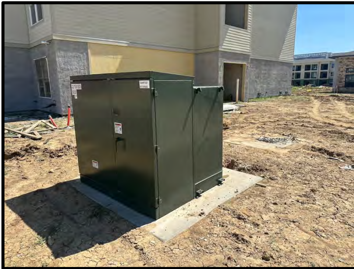
11. Installation of electrical transformers was in progress.
