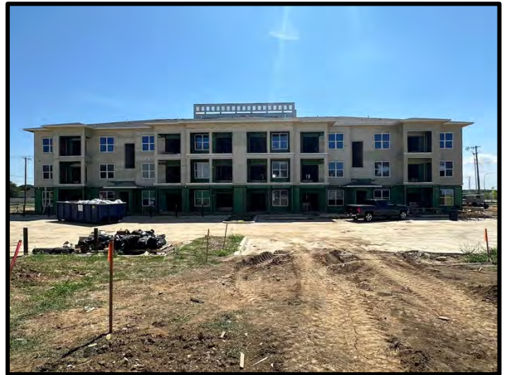
20. Exterior siding was complete at Building 6.
