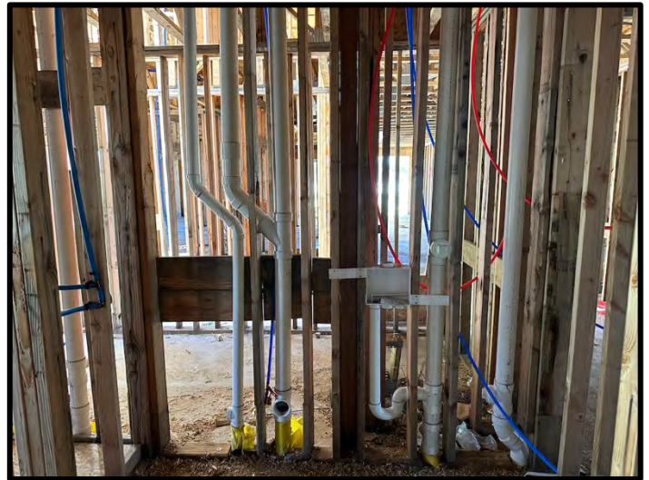
20. Plumbing rough in was in progress at Building 6.
