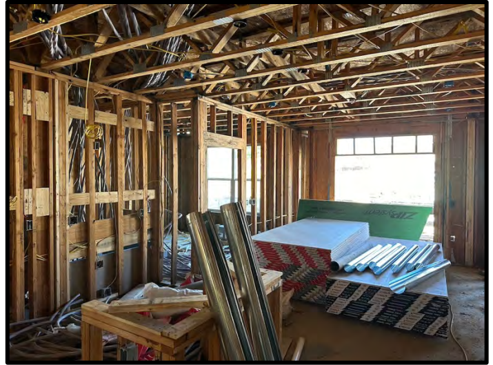
10. Vent ductwork was in progress at Building 2.
