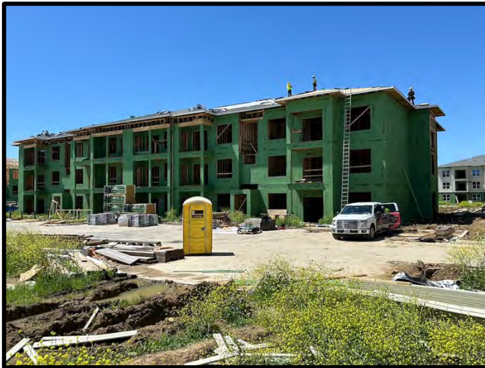
15. Exterior sheathing was complete at Building 4. Roofing was observed in progress.
