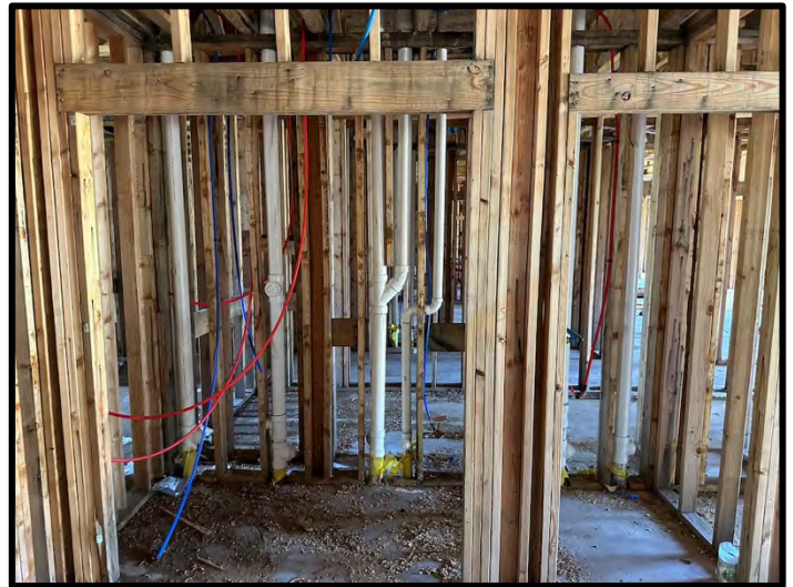
16. Plumbing rough in was in progress at Building 4.
