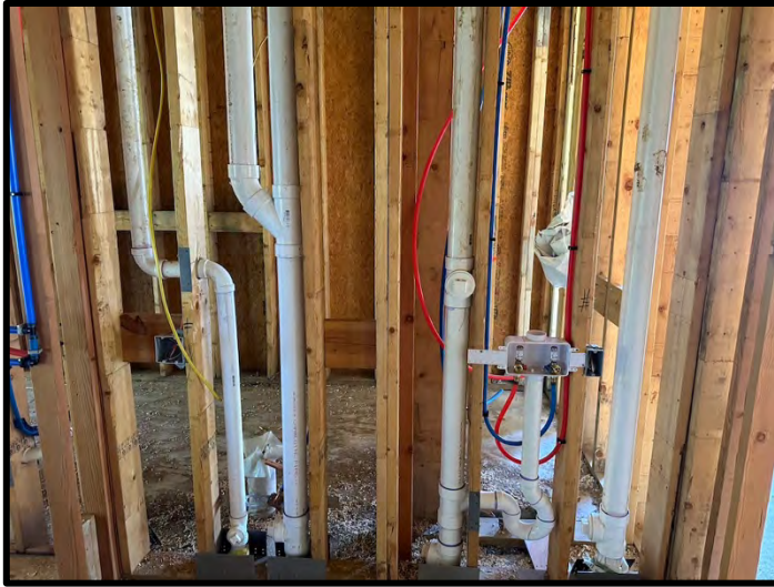
13. Plumbing rough in was complete at Building 3.
