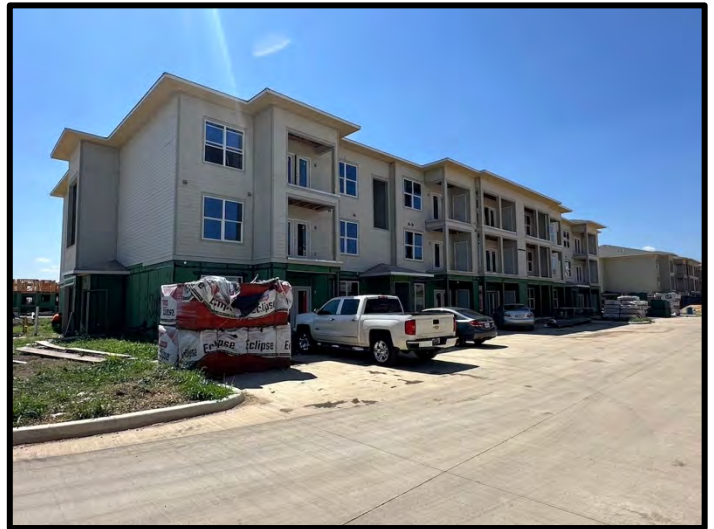
12. Exterior siding was complete at Building 3.
