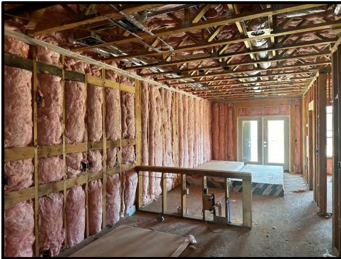
3. Unit insulation was complete at building 1.
