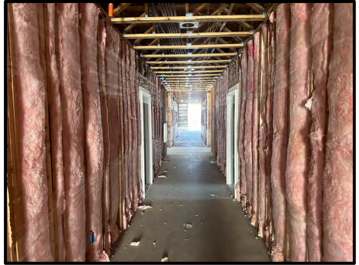
2. Breezeway wall insulation was complete at Building 1.
