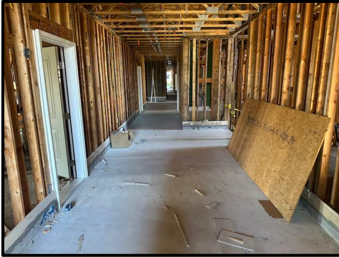
13. Breezeway lightweight concrete was complete at Building 3.
