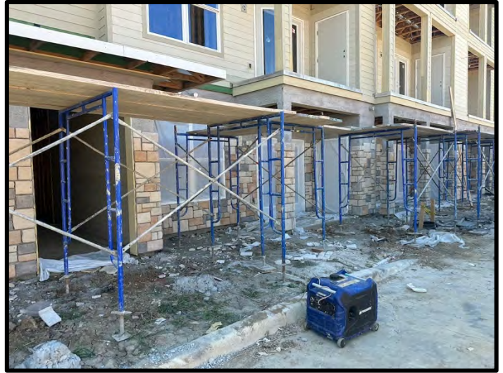
6. Stone veneer was in progress at Building 2.
