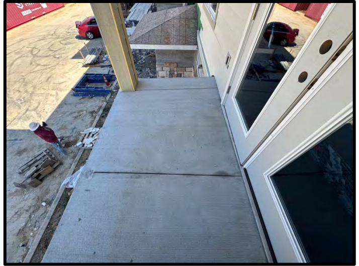
10. Lightweight concrete was complete at Building 2 unit balconies.
