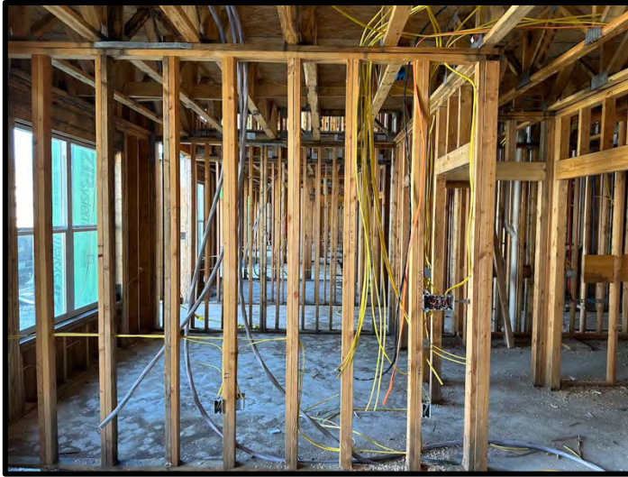
9. Electrical rough in was in progress at Building 3.
