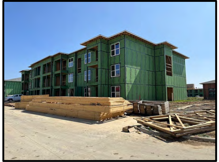
6. Windows, exterior sheathing and zip tape were complete at Building 2.
