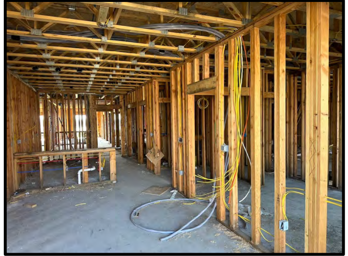
18. Electrical rough in was in progress at Building 7.
