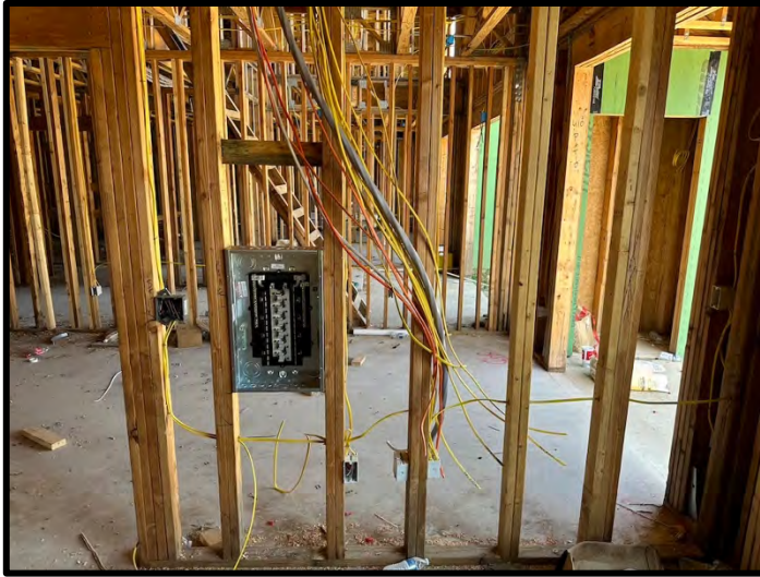
5. Electrical rough in was nearing completion at Building 1.
