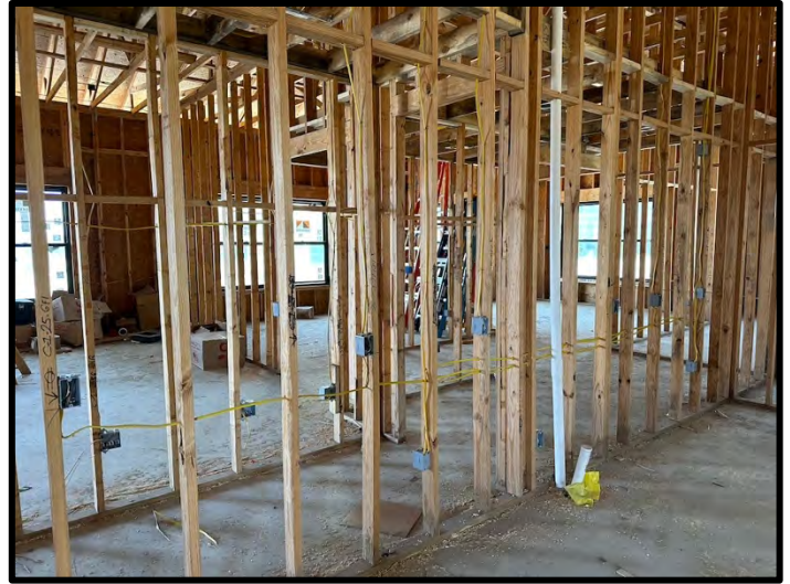
2. Electrical rough in was in progress at the Clubhouse.
