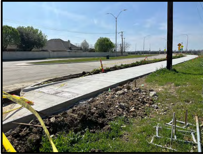
13. Concrete sidewalks were complete at Summerfields Blvd street frontage.
