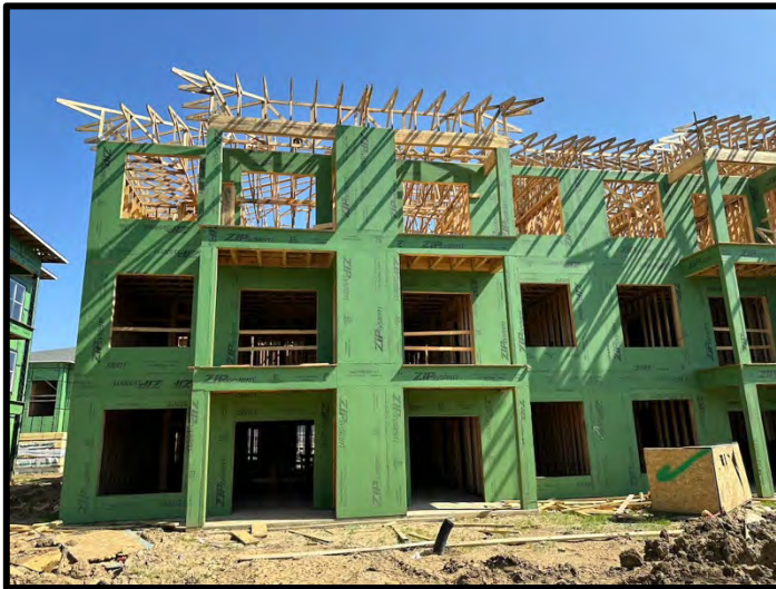
11. Roof trusses were in progress at Building 4.
