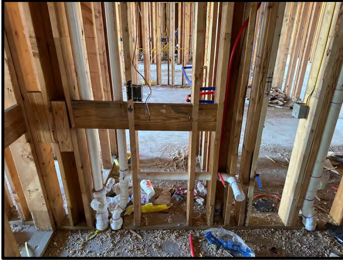
17. Plumbing rough in was complete at Building 7.
