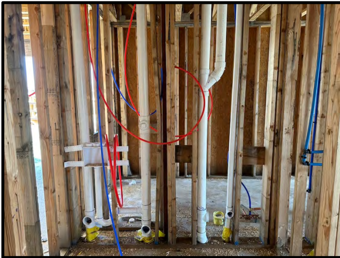
15. Plumbing rough in was in progress at Building 6.
