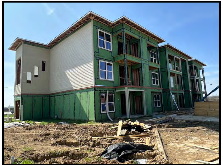
16. Exterior siding and trim were in progress at Building 7.
