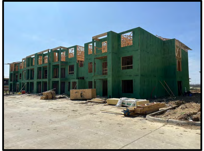
10. Framing and exterior sheathing for levels 1-3 were complete at Building 4.
