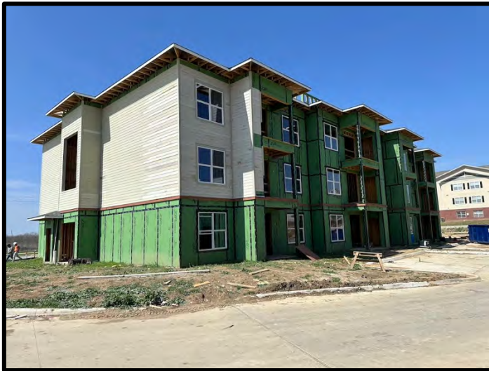
3. Exterior siding and trim were in progress at Building 1.
