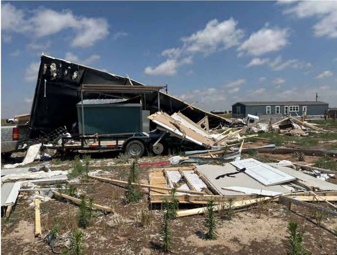
Destroyed manufactured home 4 miles west-northwest of Reese Center. The destruction was caused by a tornado Thursday evening (5 June). The image was collected by a NWS damage survey team the following day.
