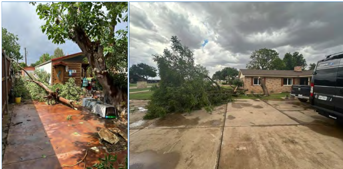
Tree damage that occurred around the Hillcrest Country Club, north of Lubbock, Monday evening. (2 June 2025). The images are courtesy of Jacob Riley.
