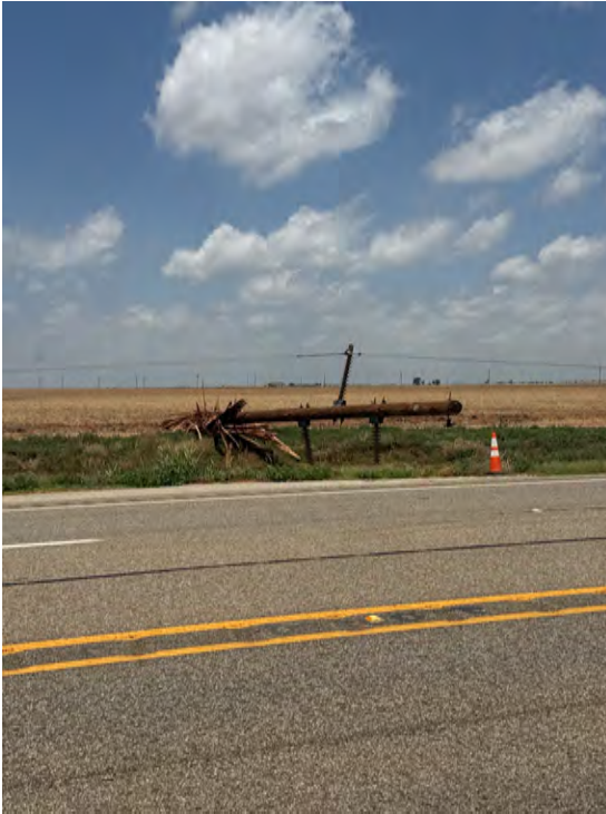
Downed power poles north of Levelland (left) and Morton (right). The damage was caused by tornadoes Thursday evening (5 June). The images were collected by a NWS damage survey team the following day.
