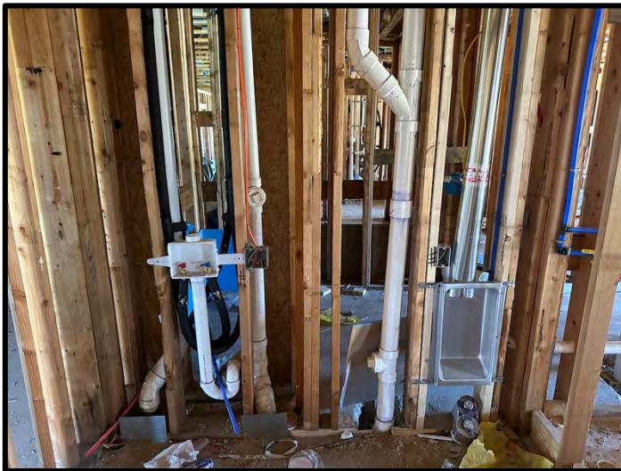
23. Plumbing rough in and dryer vents were complete at Building 7.
