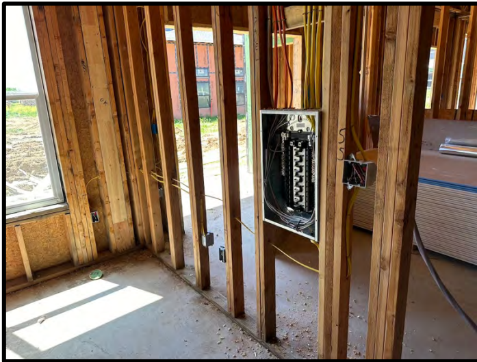
11. Electrical rough in was nearing completion at Building 2.
