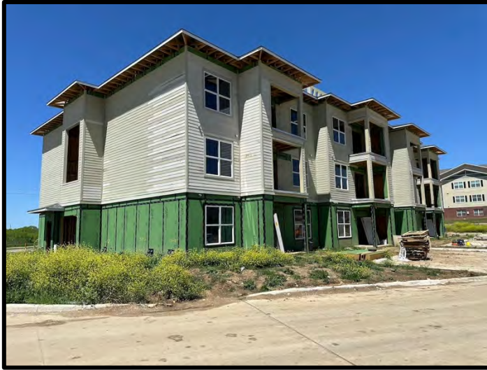
5. Exterior siding and trim were nearing completion at Building 1.
