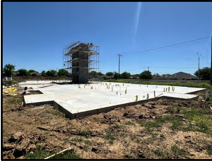
17. The concrete foundation was now complete at Building 5.
