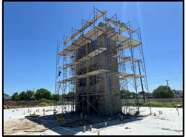
18. CMU elevator shaft was nearing completion at Building 5.
