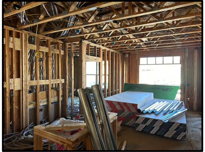
10. Vent ductwork was in progress at Building 2.
