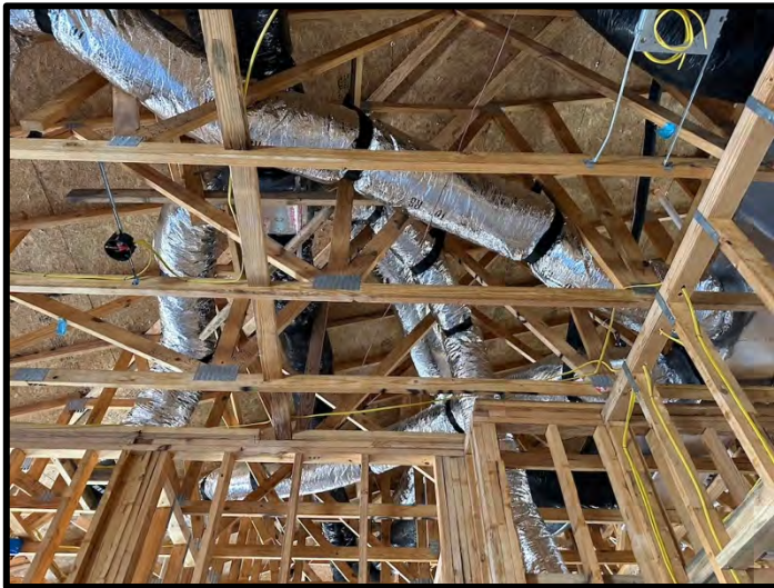
3. HVAC ductwork was complete at the Clubhouse.
