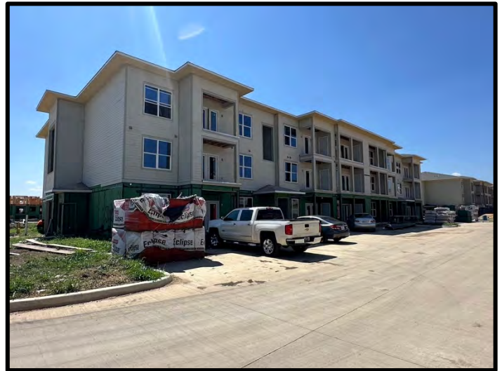
12. Exterior siding was complete at Building 3.
