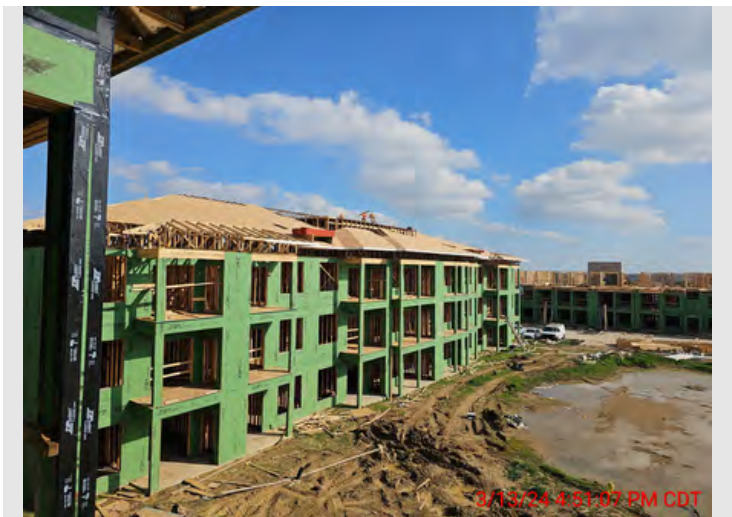
Description Installing roof decking
