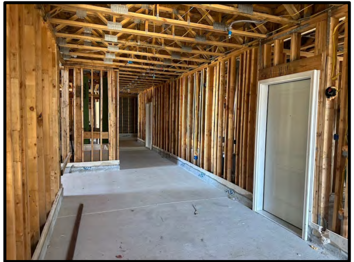
8. Breezeway lightweight concrete was complete at Building 2.
