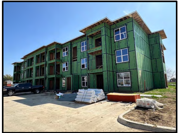
8. Windows, exterior sheathing and zip tape were complete at Building 3.
