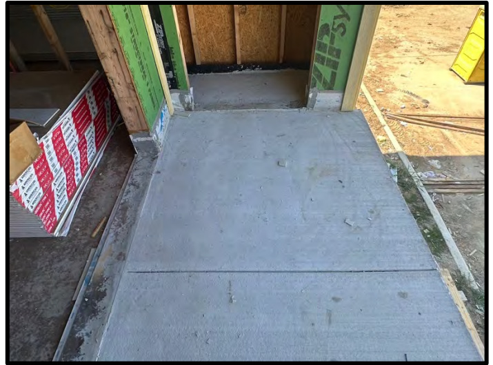
22. Lightweight concrete was complete at Building 6 unit balconies.
