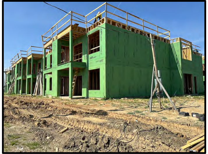
14. Re Level 2 framing was complete at Building 6. Level 3 floor decking was in progress.
