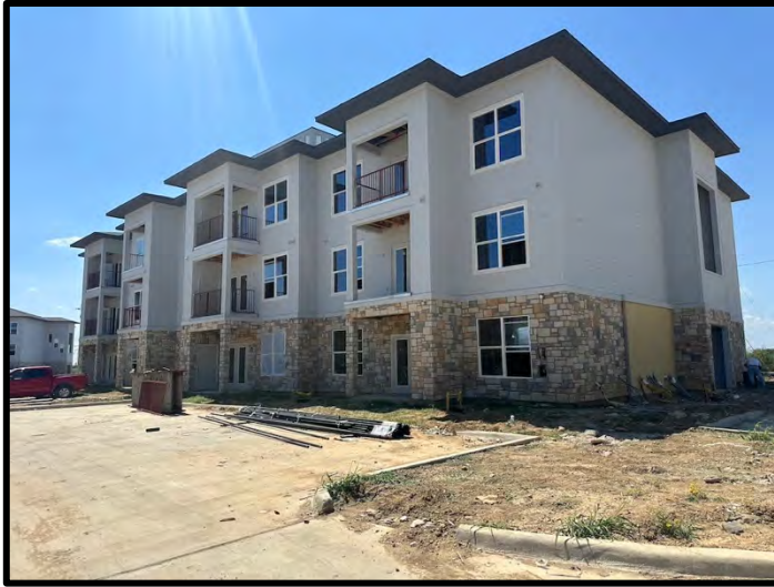
1. Exterior siding complete and balcony rails nearing completion at Building 1. Stone veneer was complete and exterior paint nearing completion.
