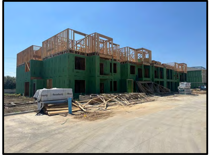
18. Framing for levels 1-2 were complete at Building 5. Level 3 framing was in progress.
