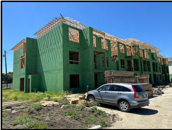
19. Level 1-3 framing was complete at Building 6. Roof trusses were nearing completion.
