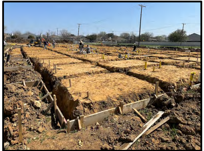
12. Re-compaction of soil and grade beams were in progress at Building 5.
