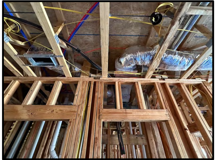
22. HVAC ductwork and refrigerant lines were complete at Building 7.
