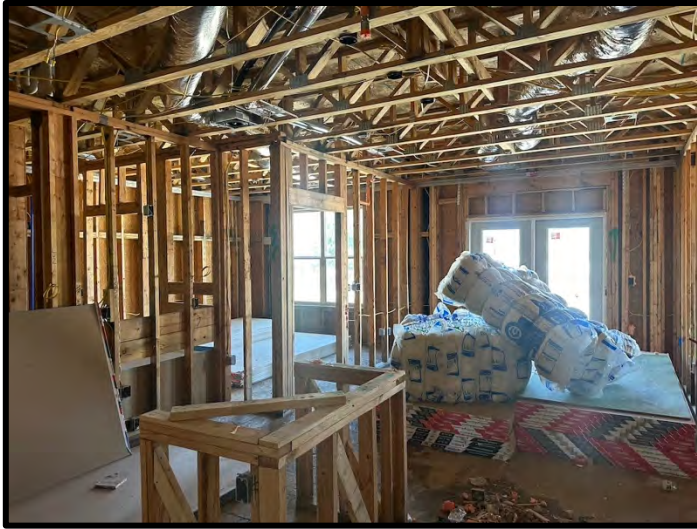
9. MEP rough in was complete at Building 2. Insulation and drywall were stored.
