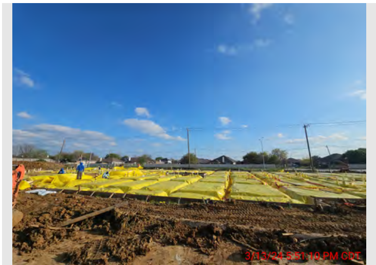
Description Installing poly
