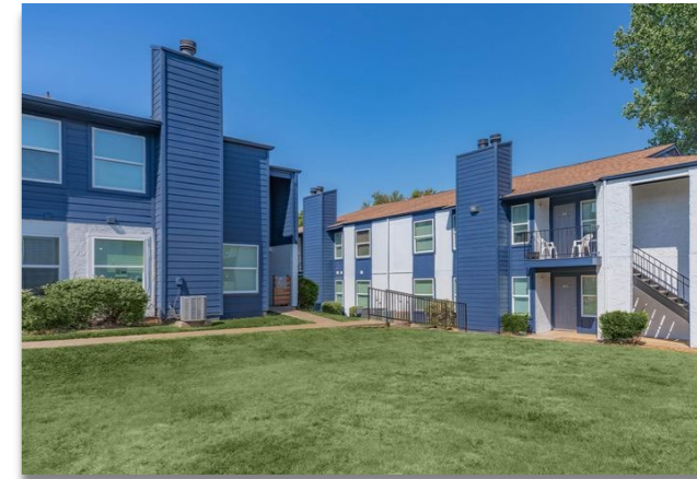
New Paint, Siding and Landscaping
