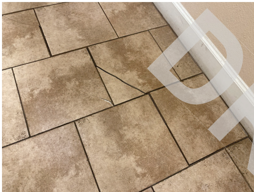
Floor tile cracking in office area from foundation settlement
