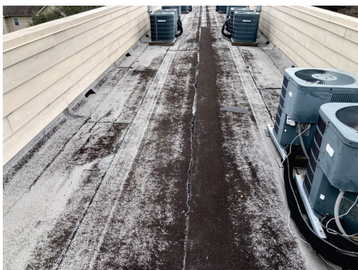
Flat, modified bitumen roofing
