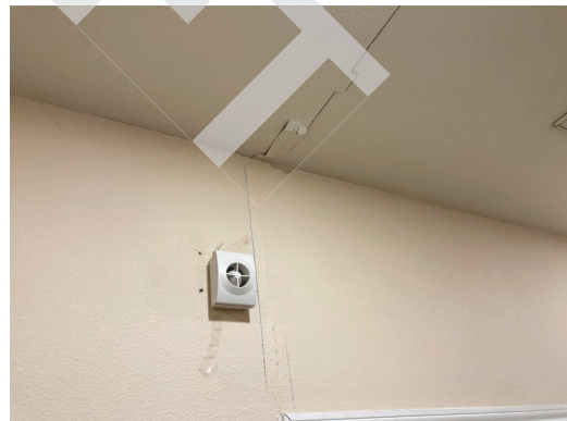
Sheetrock cracking in office area from foundation settlement
