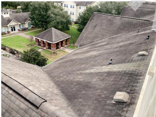
Asphalt shingle roofing
