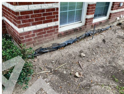
Erosion along building foundation
