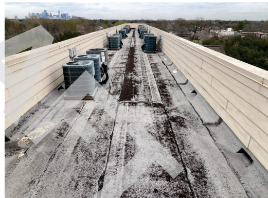
Flat, modified bitumen roofing
