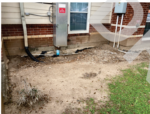
Erosion along building foundation
