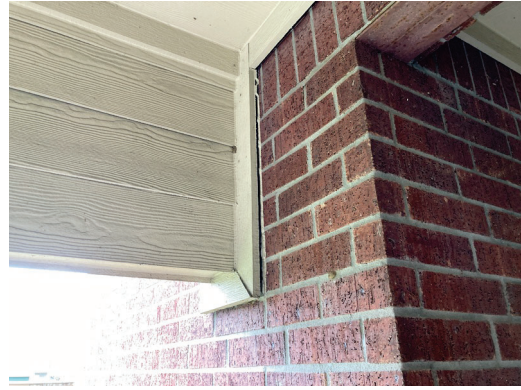
Siding separation from settlement
